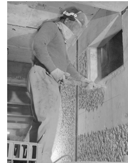
Pick and bush hammered concrete; Exposed granite aggregate
