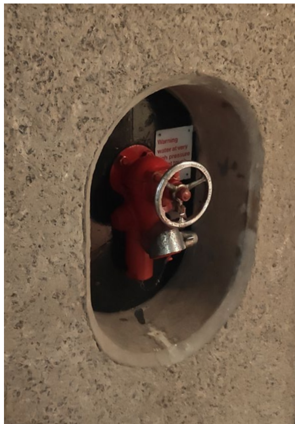
Recessed wet riser in concrete wall
