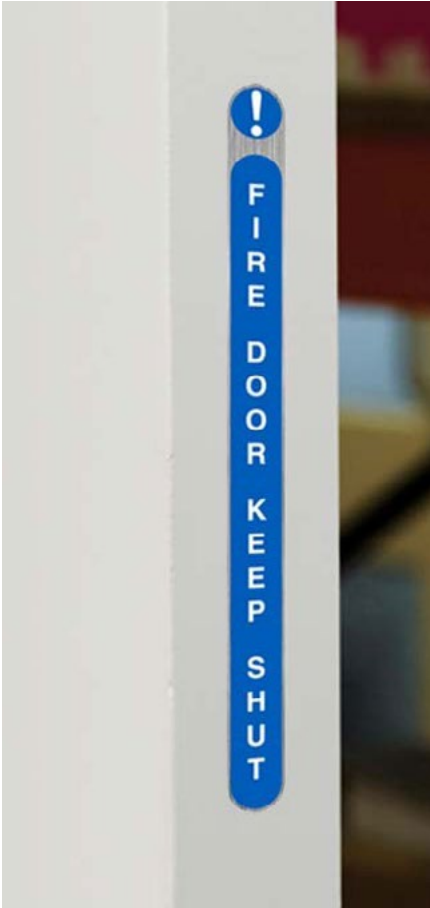
Profiling and fire signage on door leaf edge
