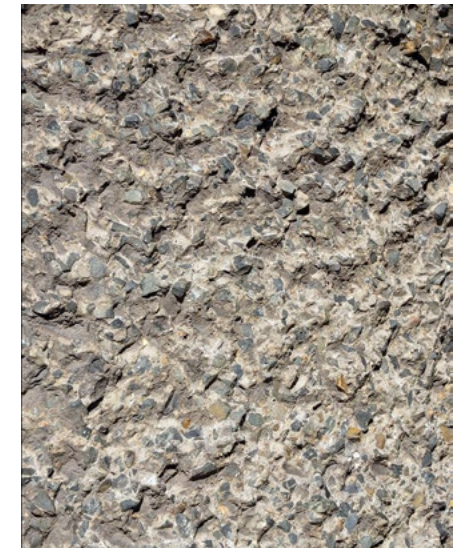
Pick and bush hammered concrete; Exposed granite aggregate
